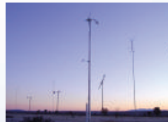
CIEMAT-CEDER test facility in Soria, Spain
