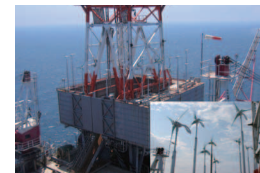
Twenty one Airdolphin Pro form an AC power micro-grid on an unmanned off shore gas rig.
